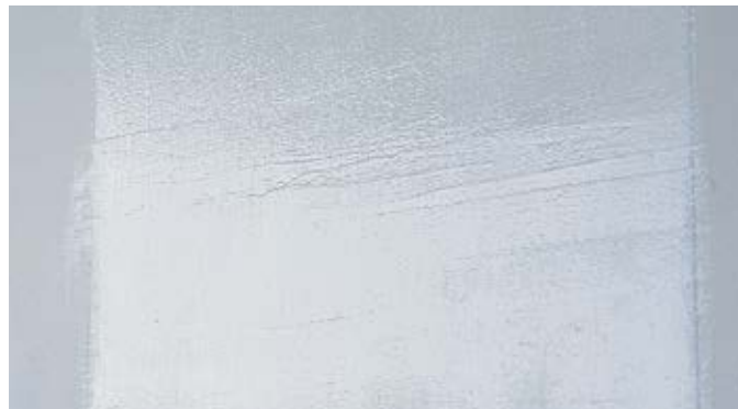
Surface finished with gloss paint
