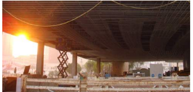
Metal framing for semi-exterior ceiling to cater for typhoons
