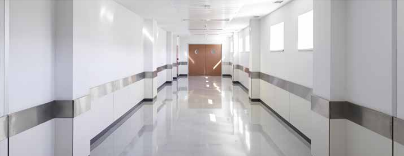
Some partitions have to be stronger and more durable than others, like this hospital corridor lined with USG Boral's abuse-resistant gypsum board.
