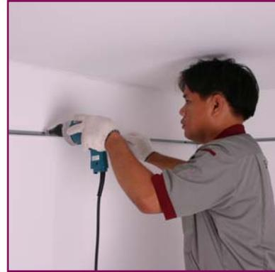
2. Fix wall angle to the wall at the desired ceiling level with screws at every 20 cm. interval, and then hang the main runner in every 121 cm. spacing, measuring from its center point.
