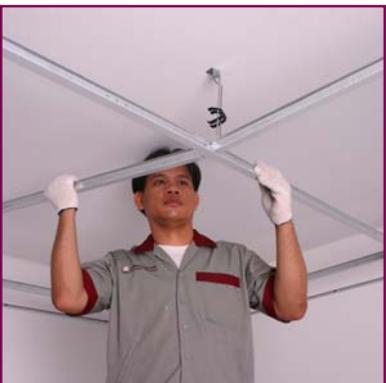
5. Insert 121 cm. long cross tee to the slot of main runner by interlock system at 60.5 cm. interval. The frame of 60.5x120 cm. will be shown.
