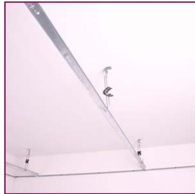
4. Hang the main runner with adjustable hanger then adjust the height of the main runner to be at the same level.
