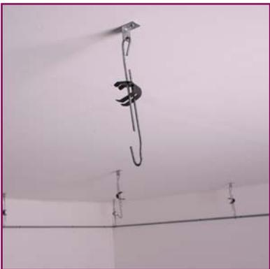
3. Attach adjustable hanger to upper floor or loft and leave 121x121 cm. spacing.
