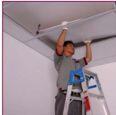
6. Lay Gypsum Ceiling Tile on the frame, then you will get T-bar Ceiling system size 60x120 cm.
