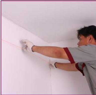
1. Determine the desired ceiling level around the room
